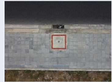
Figure 22: The drain cover is overlayed the bounding box mask
